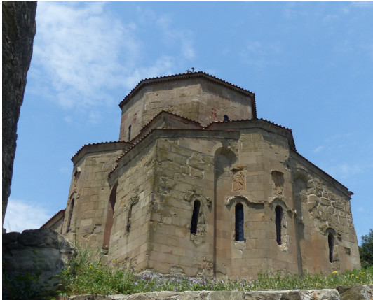
Fig. 2. Jvari from the East-south
