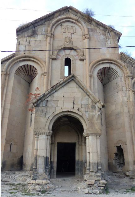
Fig. 3. Oshki's South Porch
