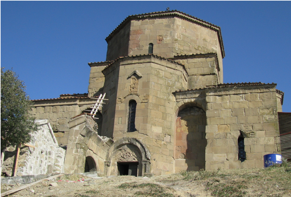
Fig. 1. Jvari Church. South façade. 2
