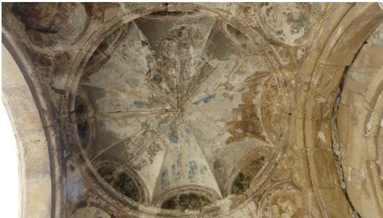
Fig. 16. Bagrat'i. South Porch with Umbrella Cones' Dome.
